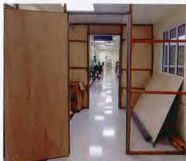
The picture shows the construction of the anteroom connecting between the Phase 1 and Phase 2 of GICU.
