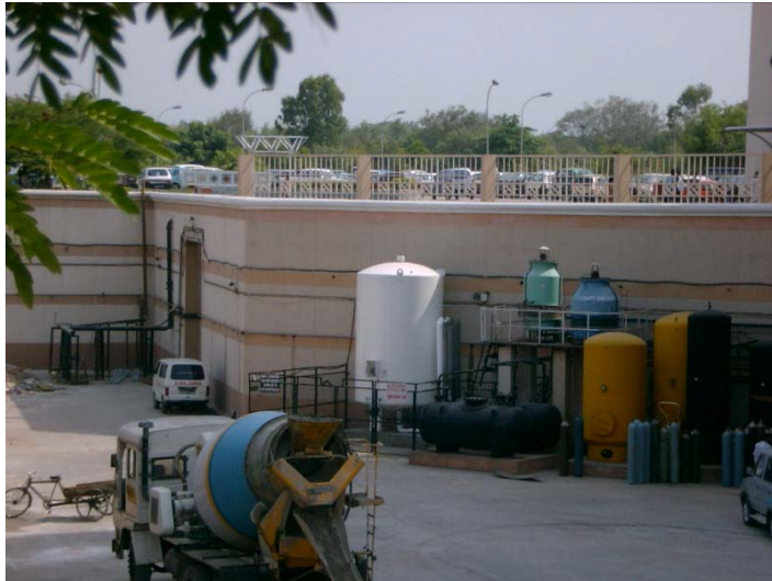
Air and Oxygen Banks in the basement
