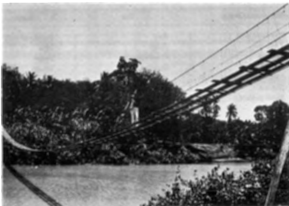
Fig. 37 View of suspension bridge linking Kampung Labuaya to Tuaran town-ship.
